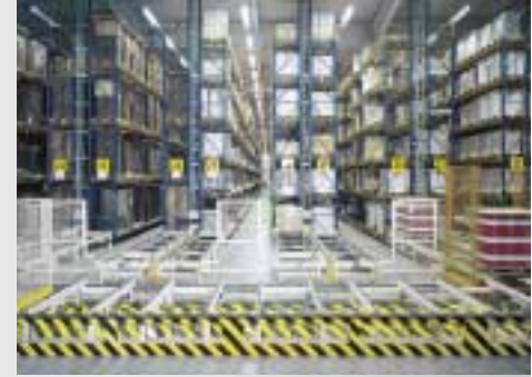
Pallets from material storage that have to be dispatched are moved to a shuttle using the conveying system.
