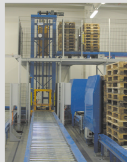
Vertical conveyor and empty pallet checking station
