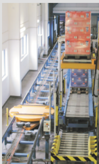
Complex conveying system in one of the connecting bridges
